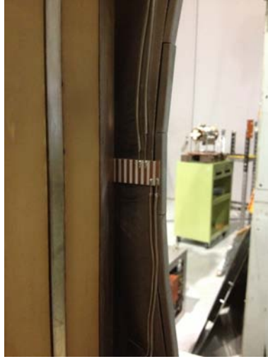
Figure 5.4: Electrostatic probe array installed on the inner wall of the private limiter.
