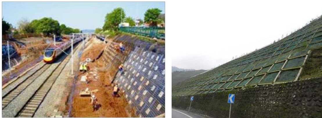
Figure 1.1: Typical landslide protection works; (a) along railway tracks (FHWA, 2003), (b) along highways (Hongbai county, Wenchuan, China)
