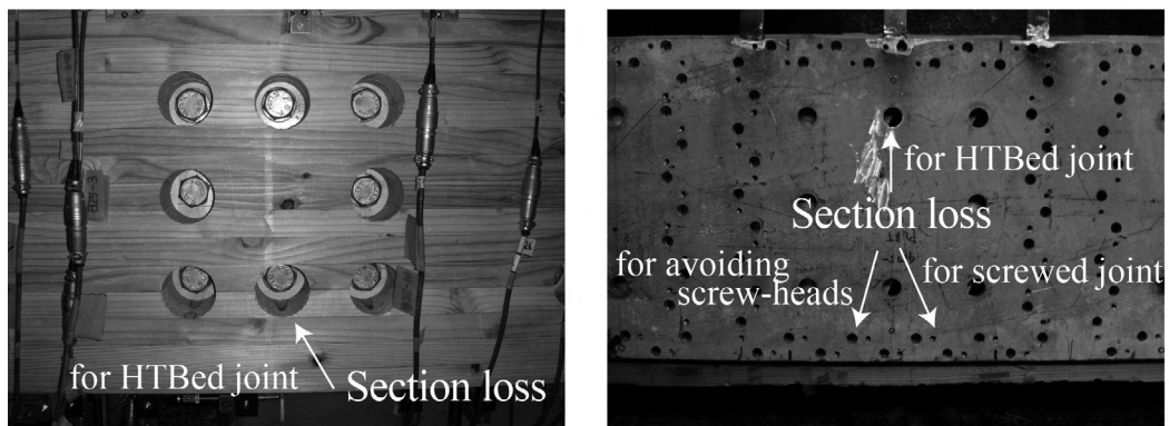
Fig. 3.17. Section loss of pre-drilled holes
