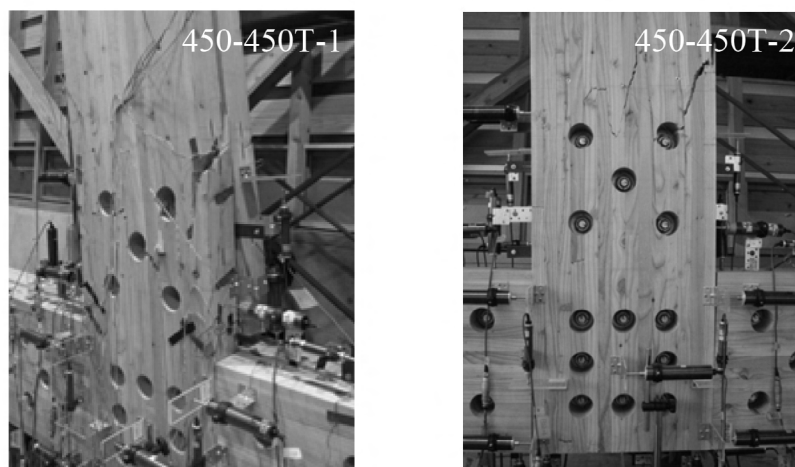
Fig. 3.34. Bending fracture at joint end
