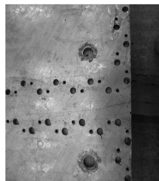
Fig. 3.52. Bending deformation of pre-drilled hole in steel
