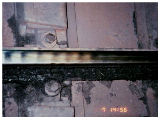
(b)防振まくら木道床, 171mR, \lambda=46\text{-}50\text{mm} V=45\text{km/h} , f=250\text{-}270\text{Hz}
