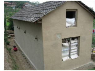
(c) PP-band mesh retrofitted building after completion
