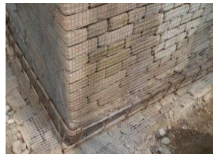
(b) Jacketing by galvanized wire mesh
