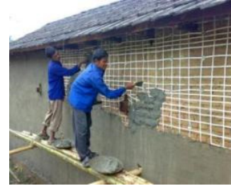
(b) Mud plaster work after PP-band mesh installed
