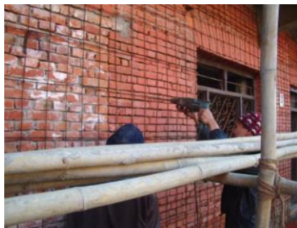
(a) Jacketing by reinforced concrete mesh
