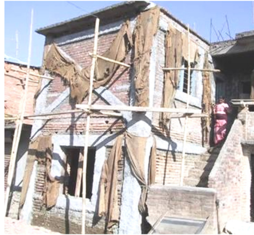
(c) Building after second layer of concrete retrofitted by splint-band system
