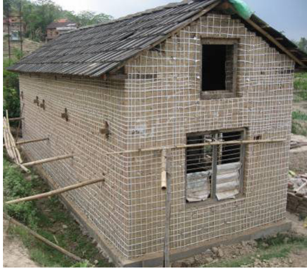
(a) Low strength masonry building after installation of PP-band mesh
