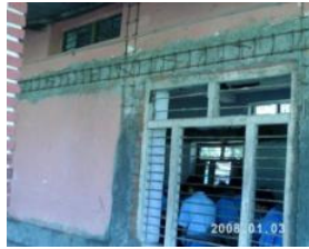
(a) Building under retrofit by splint-bandage method
