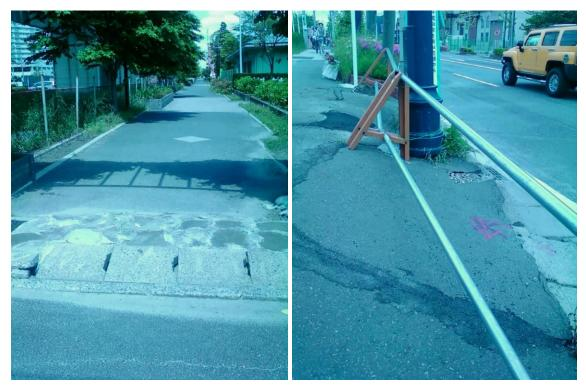
**Figure 2.12. Liquefaction on the streets**
