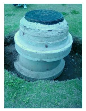
Figure 2.15. Floating of manholes
