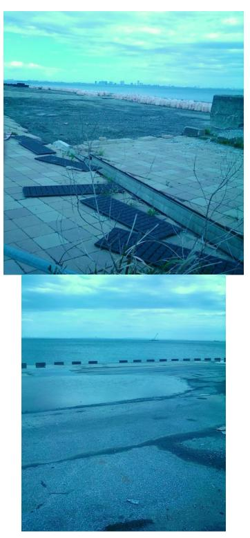
Figure 2.14. Liquefaction in the harbor area
