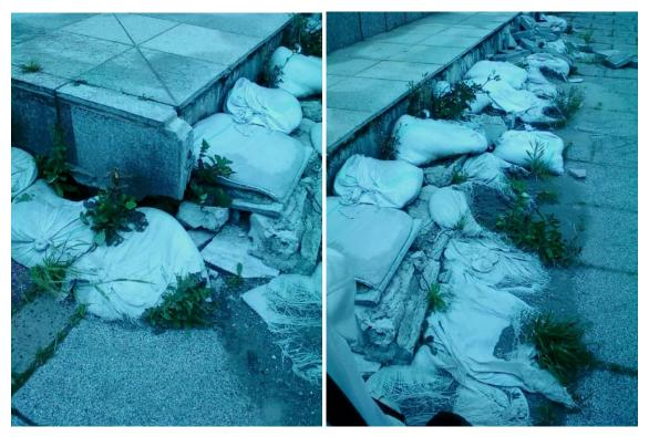
Figure 2.10. Differential settlement observed around the City
