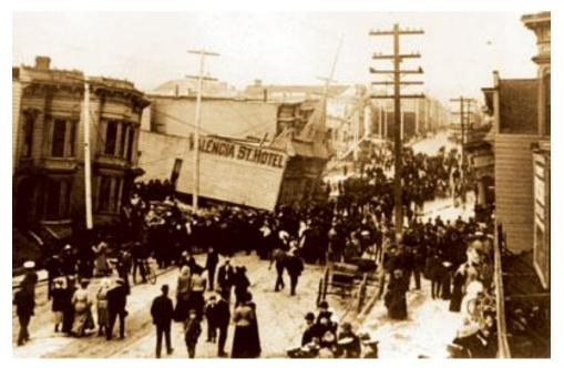
**Figure 2.2. Liquefaction in the Valencia Street Hotel**<sup>2</sup>
