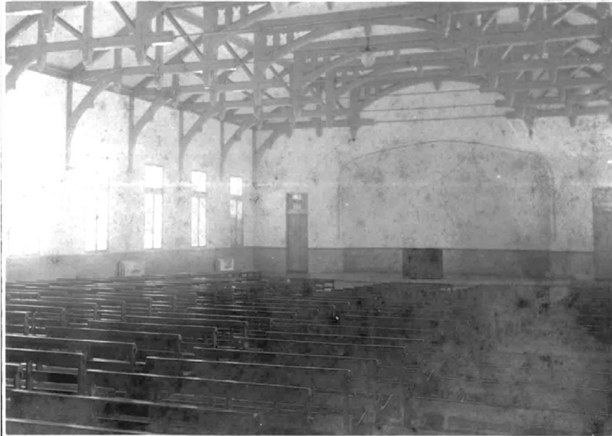
Figure 3-24 The Wooden Truss of The Auditorium
