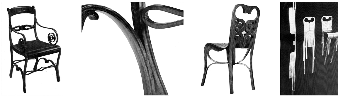
Fig. 2.3.9 Thonet's early experiments with laminated veneer furniture, from left to right: A chair dating between 1836-40 and its detail of the leg composed of glued bent veneers, 83 experimental chair from laminated veneers from 1880 and a scale model showing its construction. 84
