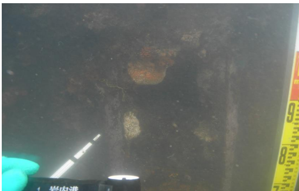
Fig.2-32 腐食孔
