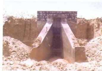
Damaged sluice
