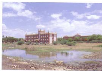
Encroachments by Government buildings
