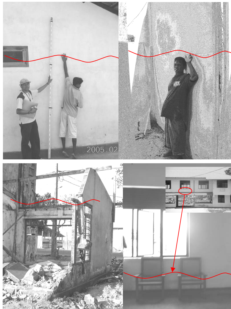
Fig 3.2: Inundation heights identified by watermarks left in the walls, damaged buildings
