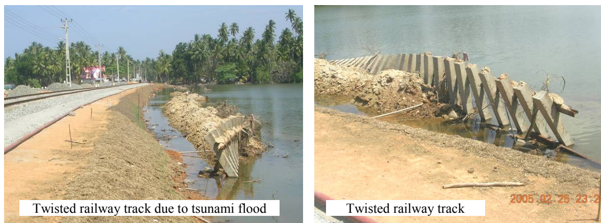
Fig 3.14: Damages in Kosgoda railway track.
