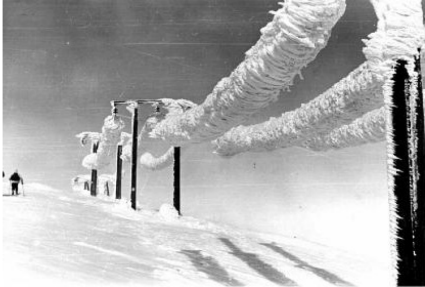
Fig.1-3 Icing on utility poles and power cables (2)
