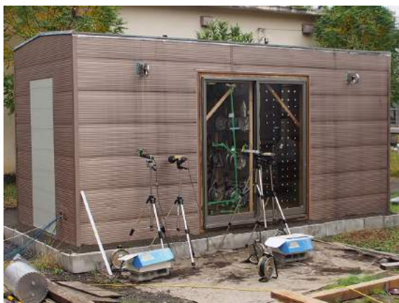
Fig. 4.1: The test house for experiment.
